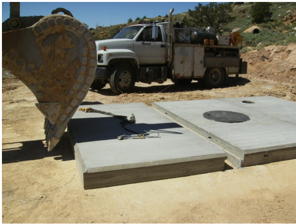
Placement of Sheep II Shaft cap with locking manhole access.
