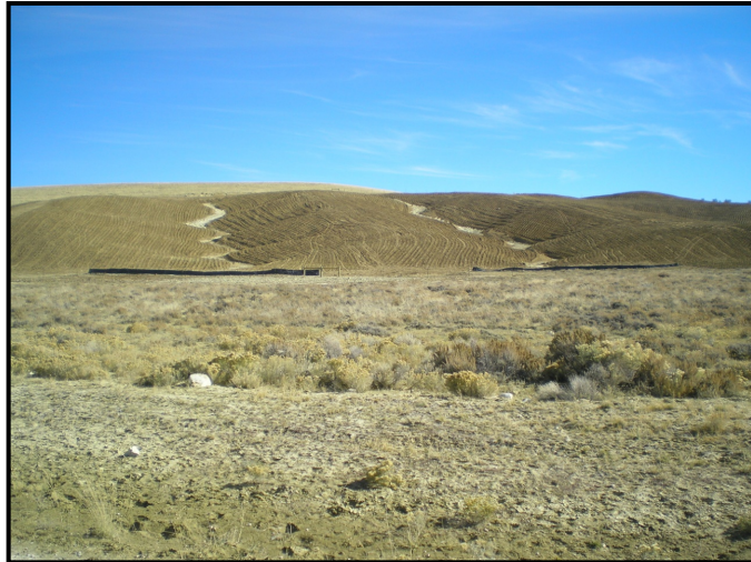
AERIAL VIEW OF THE COMPLETED STEEP SLOPE NATURAL REGRADE IN FOREGROUND – TRADITIONAL 4:1 RECLAMATION SLOPES WITH CONTOUR DITCHING IN DISTANCE
