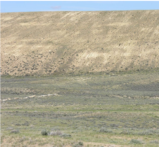
AERIAL VIEW OF THE COMPLETED STEEP SLOPE NATURAL REGRADE IN FOREGROUND – TRADITIONAL 4:1 RECLAMATION SLOPES WITH CONTOUR DITCHING IN DISTANCE
