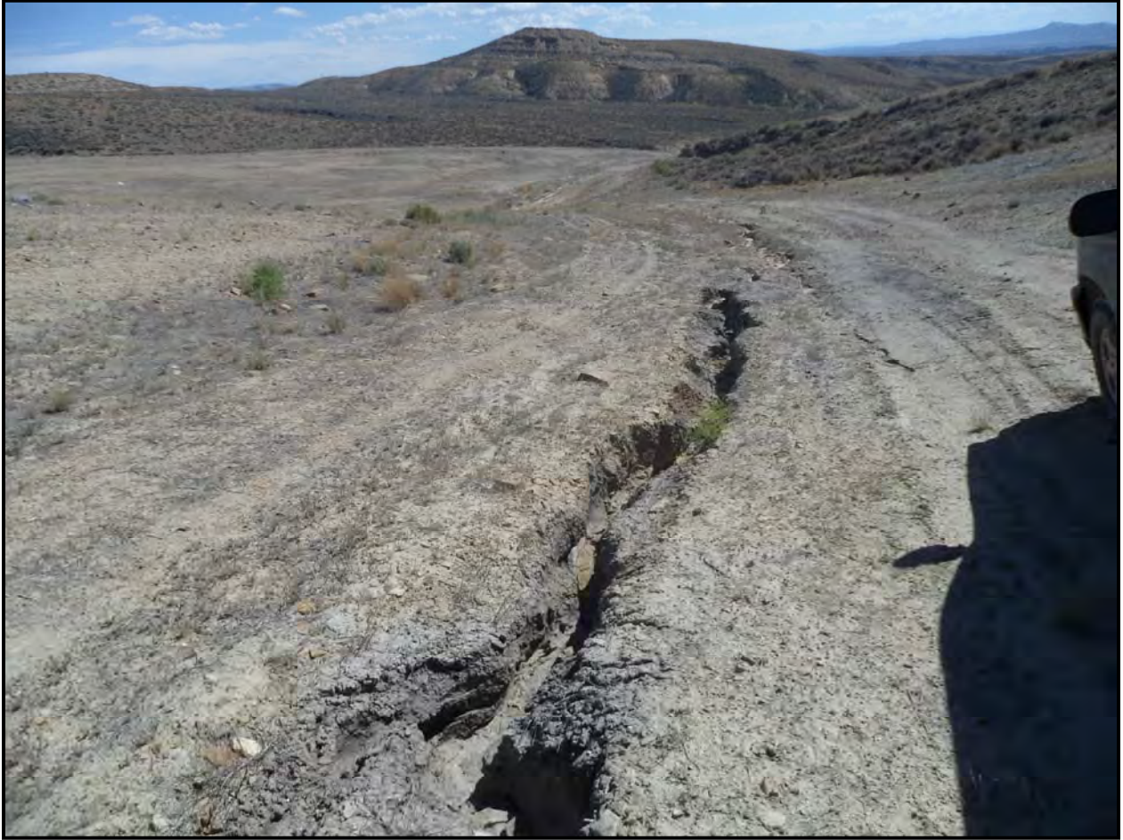
Figure 9: Traditional Channel Main: Failure in August 2013, Looking Downstream
