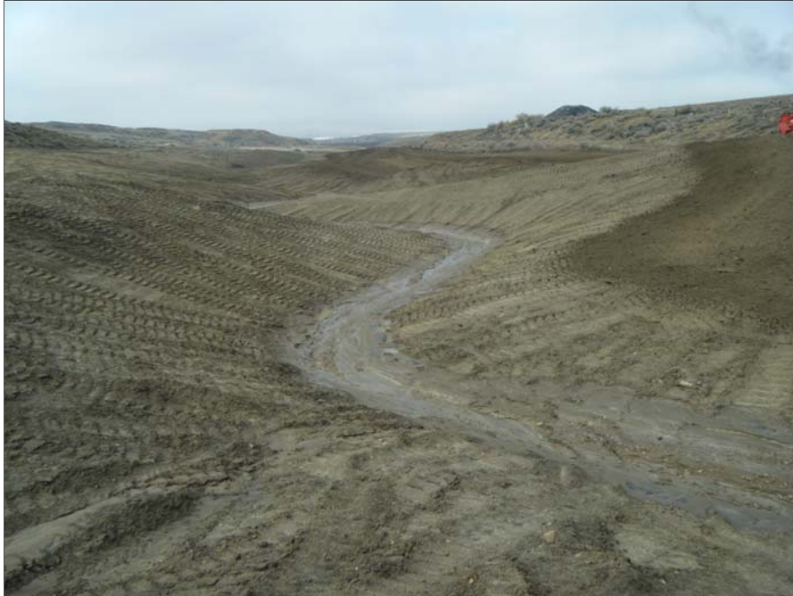
Figure 22: Freshly Constructed Lionkol Channel Following High Runoff Flows
