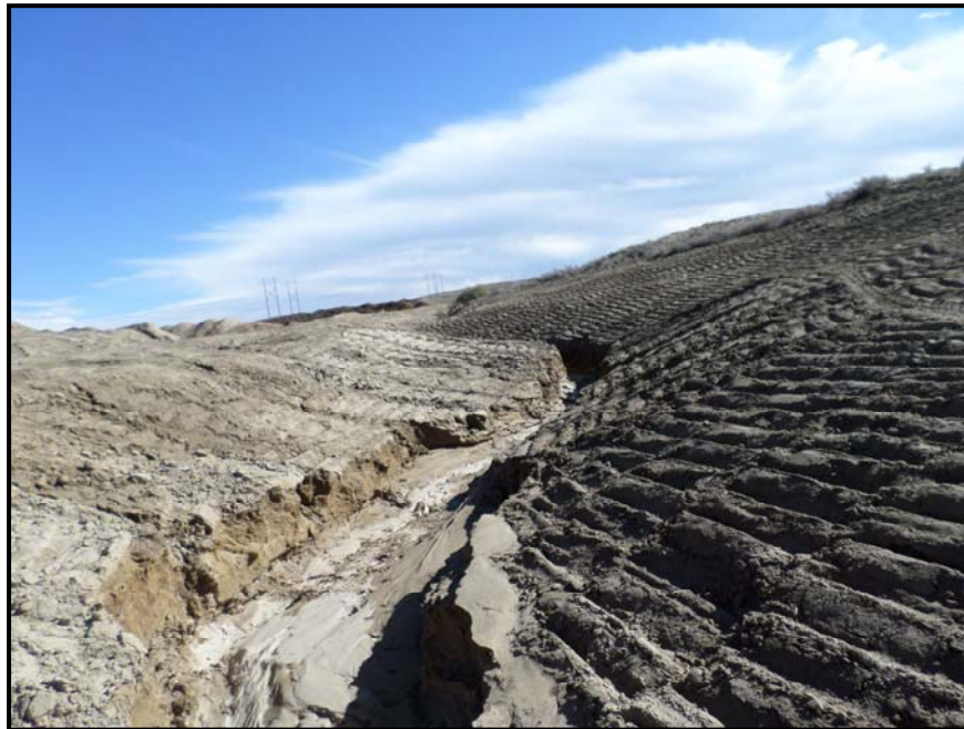
Figure 26: Lionkol West Drainage Upper Main During Construction, Channel Failure
