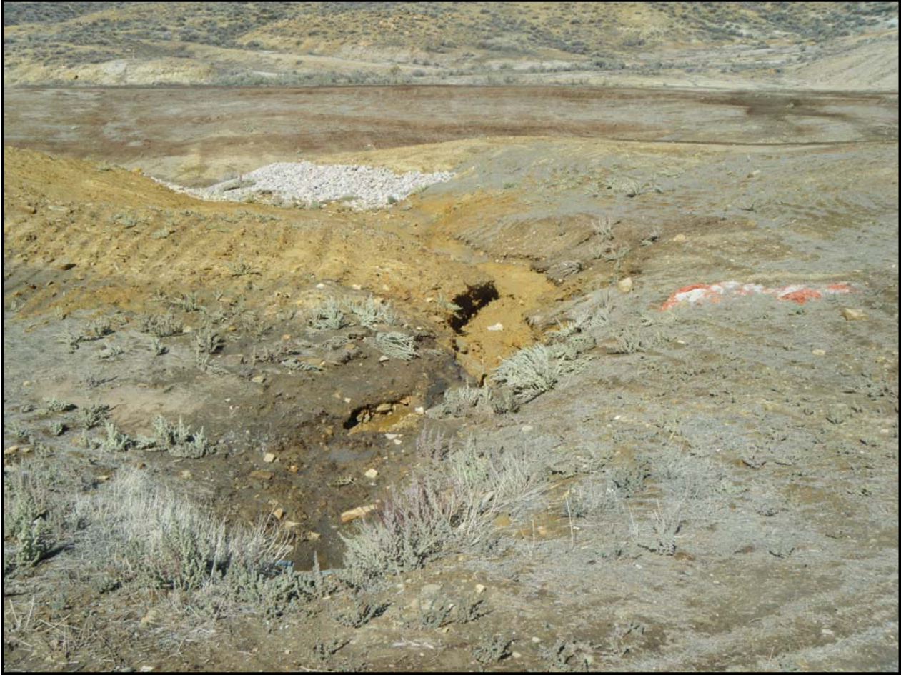
Figure 23: Lionkol Upper Main Drainage: Tributary L1 Failure Upstream of Rock Structure.
