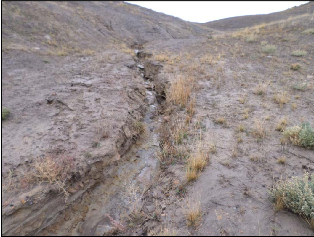
Figure 19: Lionkol North Main: Channel failure incised to bedrock
