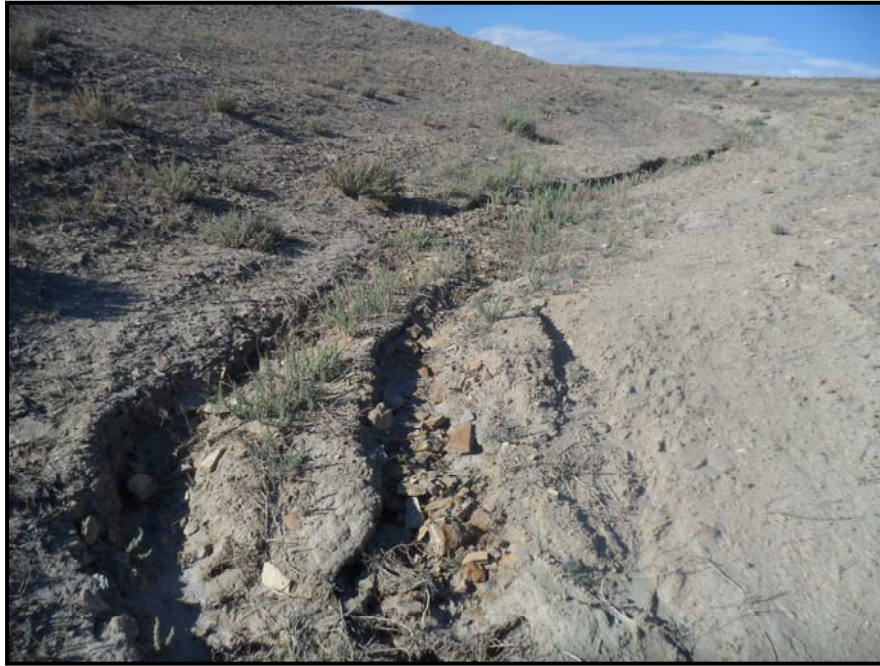
Figure 17: Reliance No. 3 North Spoils Main Failure: Channel cutting through point bar
