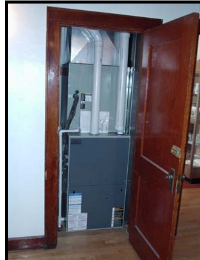
New Heater and Air Conditioner:
