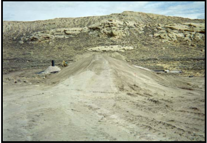
Completed Attenuation Feature with Outlet Structure:
