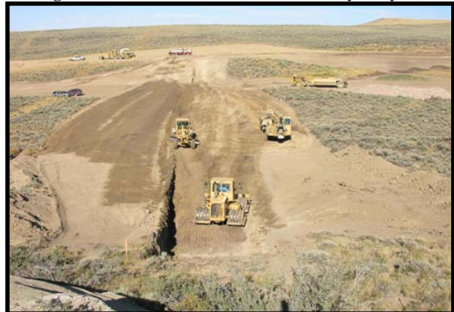
During Construction – Construction of Key Way
