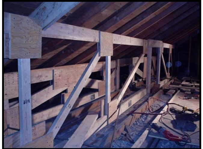
Structural Trusses Constructed to Reinforce Roof:
