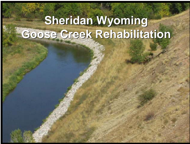
Rip Rap Protected Bank
