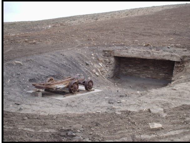
Restored Portal, Kemmerer
