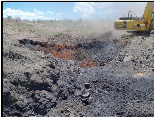
Coal Fire Excavation, Kemmerer
