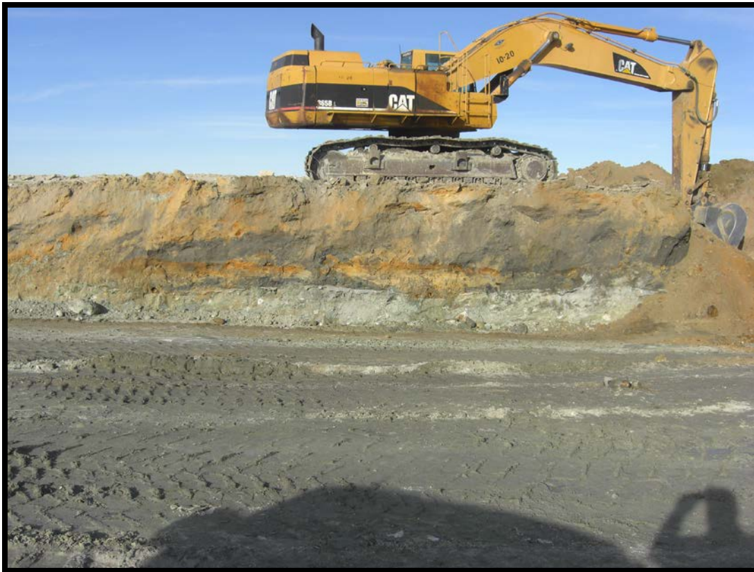
Excavation of spent ore materials in the Western Nuclear heap leach facility, Phase 1. Note the color change to light gray in the lower portion of the excavation, with pieces of liner visible at the heap contact.
