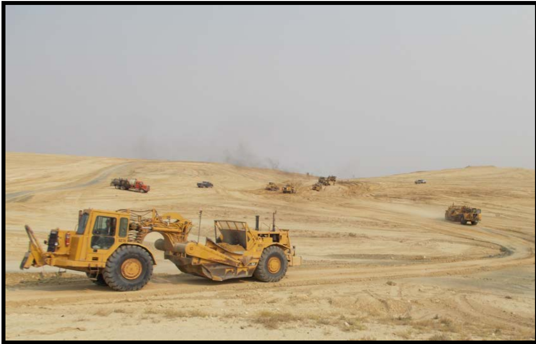
GPS Equipped Scraper Assisted by GPS dozer and a Fleet of Conventional Scrapers Constructing an "A" Channel on the North Loco Spoils, Phase 3. Completion of this Project Anticipated for Fall 2012.
