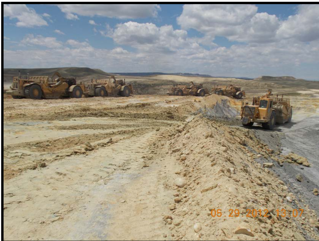
Excavation of Unsuitable Materials at the Loco Spoils during Phase 2.
