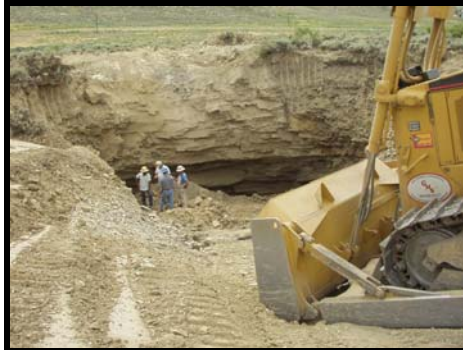
Excavation in progress
