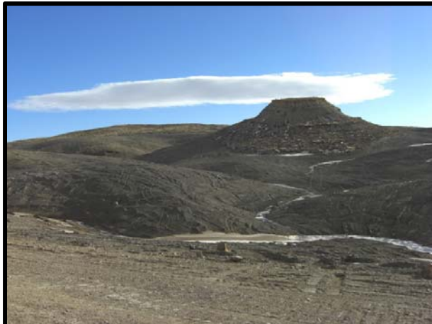
Completed Natural Regrade Channel
