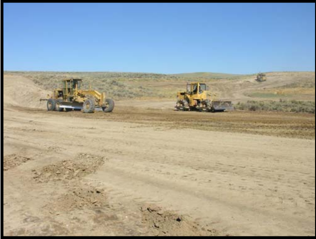
During Construction – Compaction of Earthen Structure
