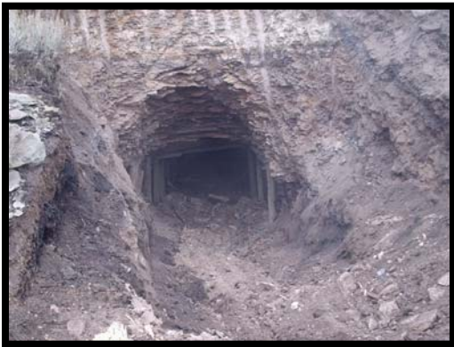
Excavated Portal (to competent roof and back)
