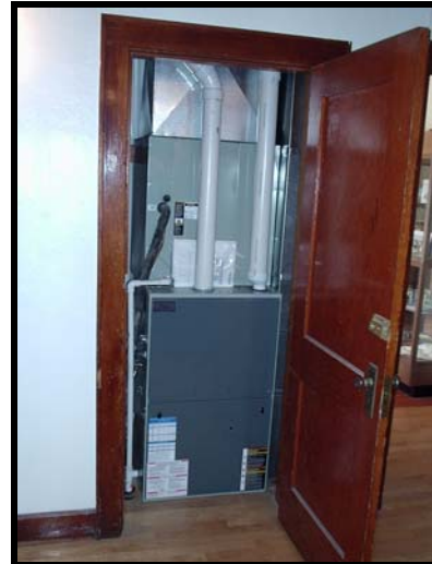
New Heater and Air Conditioner:
