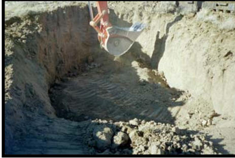
Compaction of Backfill
