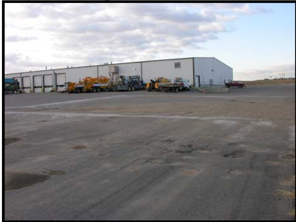
Macy's Truck Stop Subsidence:
