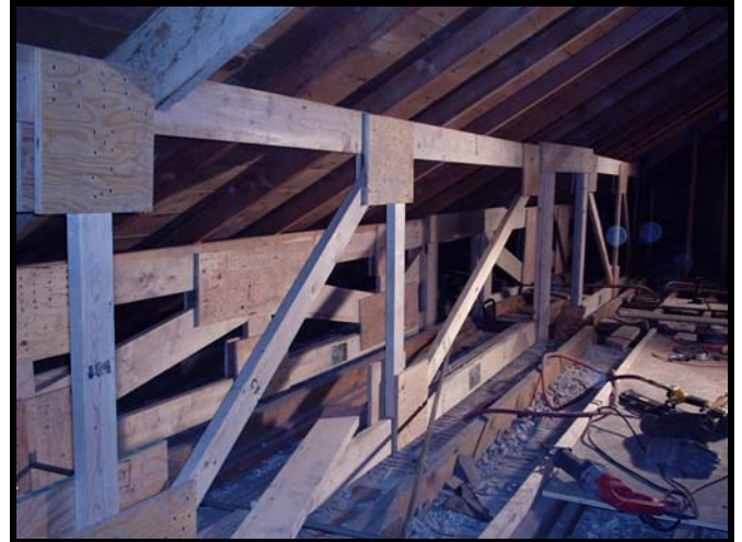
Structural Trusses Constructed to Reinforce Roof:
