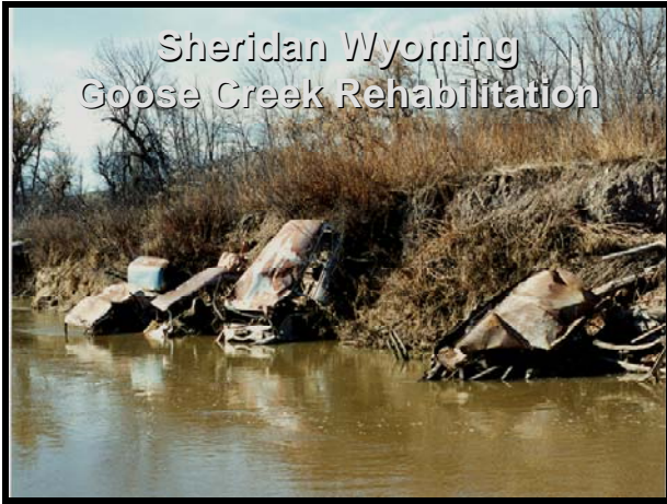
“Wyoming Rip Rap”
