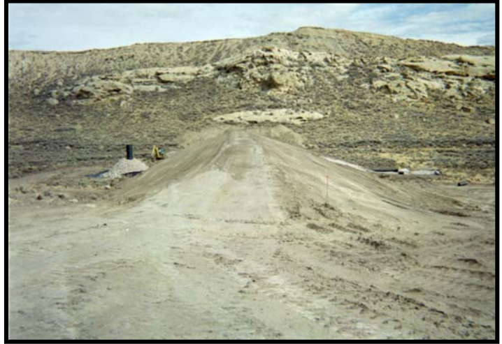
Completed Attenuation Feature with Outlet Structure:
