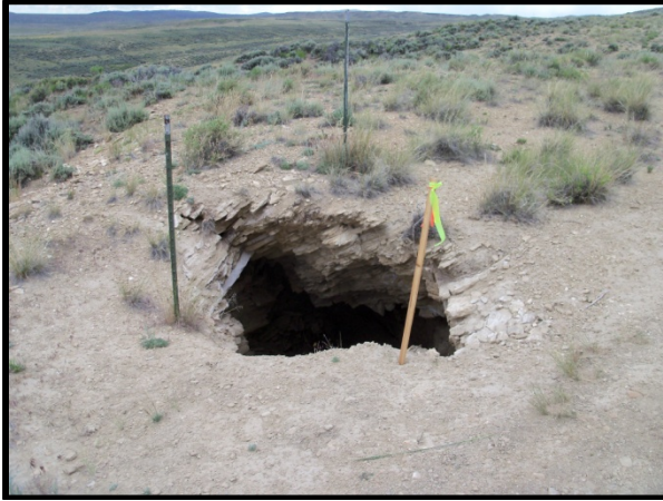
Open Subsidence, Glencoe Site, Kemmerer
