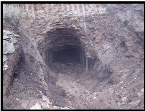
Excavated Portal (to competent roof and back)
