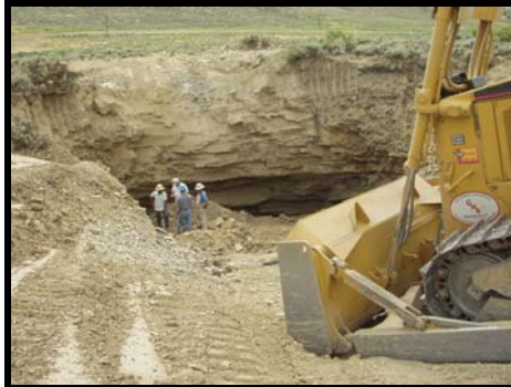
Excavation in progress
