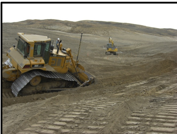
Channel Construction for Natural Regrade Design
