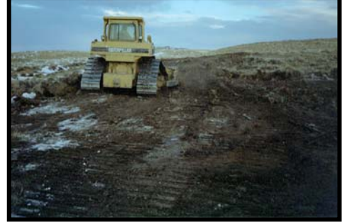
Topsoil Replacement/Grading
