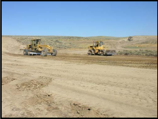
During Construction – Compaction of Earthen Structure
