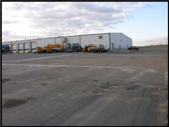
Macy's Truck Stop Subsidence:
