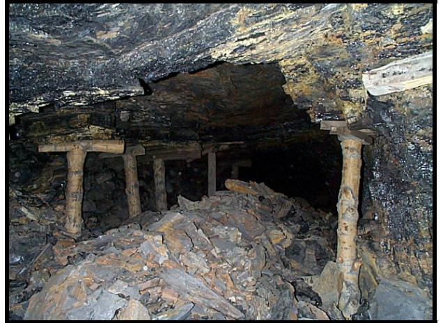
Hot Springs County Open Portal:
