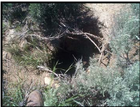
Open Subsidence >35 Feet Deep
