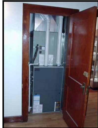
New Heater and Air Conditioner:
