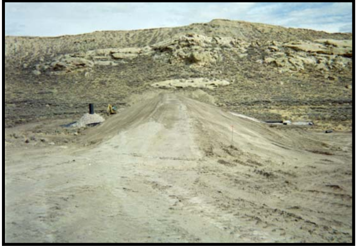
Completed Attenuation Feature with Outlet Structure:
