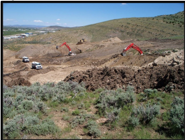
Large Scale Excavation, Evanston Area
