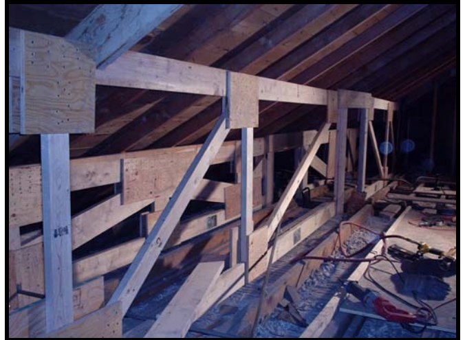
Structural Trusses Constructed to Reinforce Roof:
