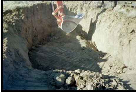
Compaction of Backfill
