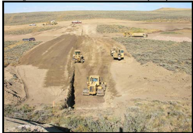
During Construction – Construction of Key Way
