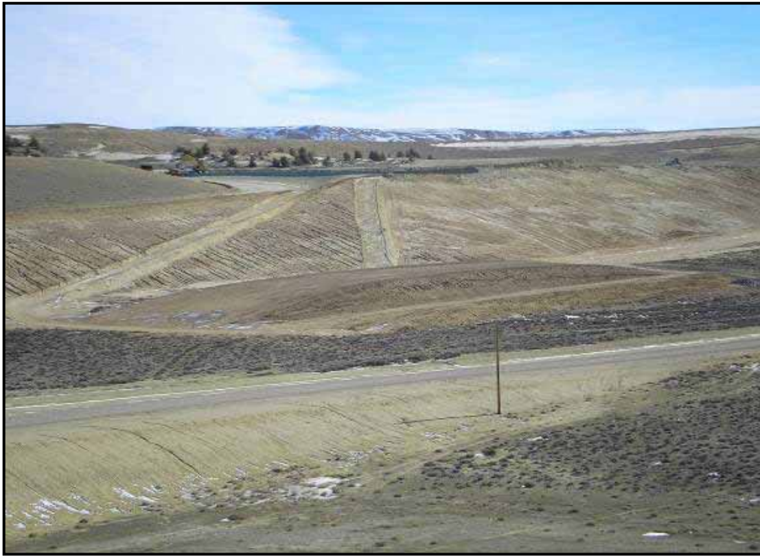
Photo 2: Central Spoils prior to reclamation. Note long, continuous, eroded 3:1 slope
