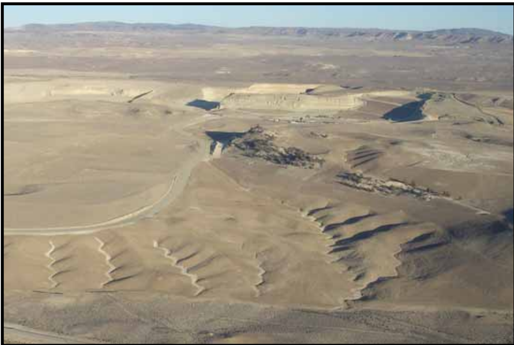
Photo 10: Aerial view of the completed project with D9 and K Pit highwalls visible in the background
