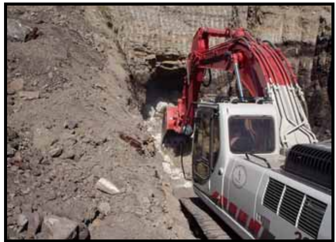
Photo 18: Typical grouted rock bulkhead installation
