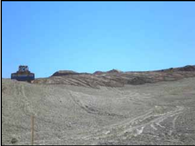
Photo 6: Dozer spreading coversoil on ridge line
