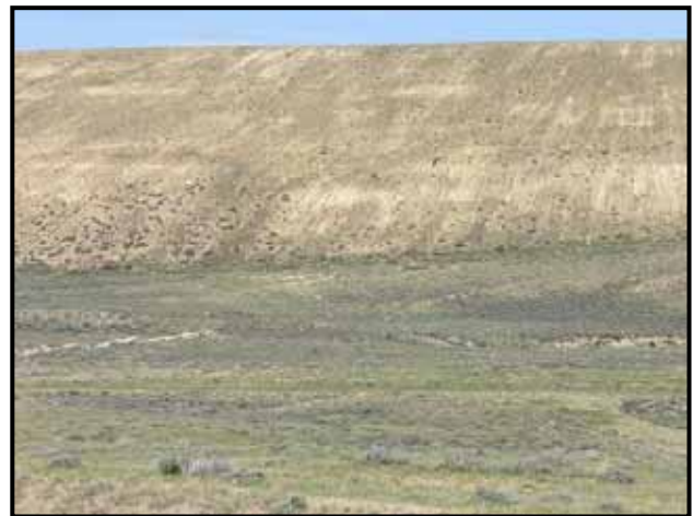
Photo 8: View from the county road of eroding 3:1 slope before reclamation
