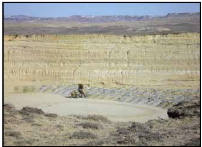
Photo 3: Placement of backfill in the K Pit
