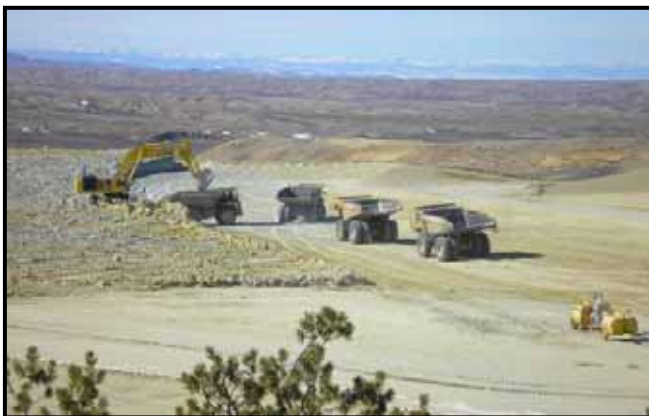
Photo 4: Bulk Haulage from Central Spoils to the K Pit
