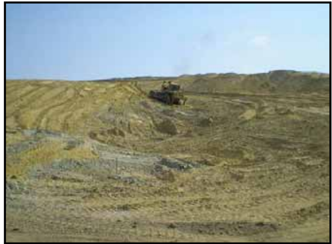
Photo 5: Dozer equipped with machine control GPS shaping an "A" channel
